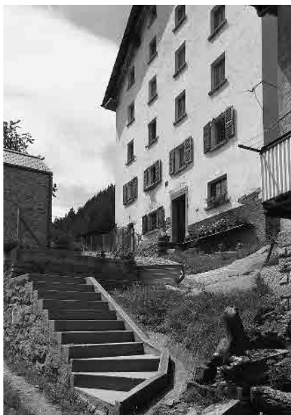
2 Dimora in muratura, 1868
