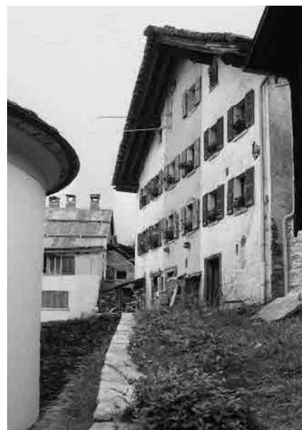
10 Dimora in muratura, 1878
